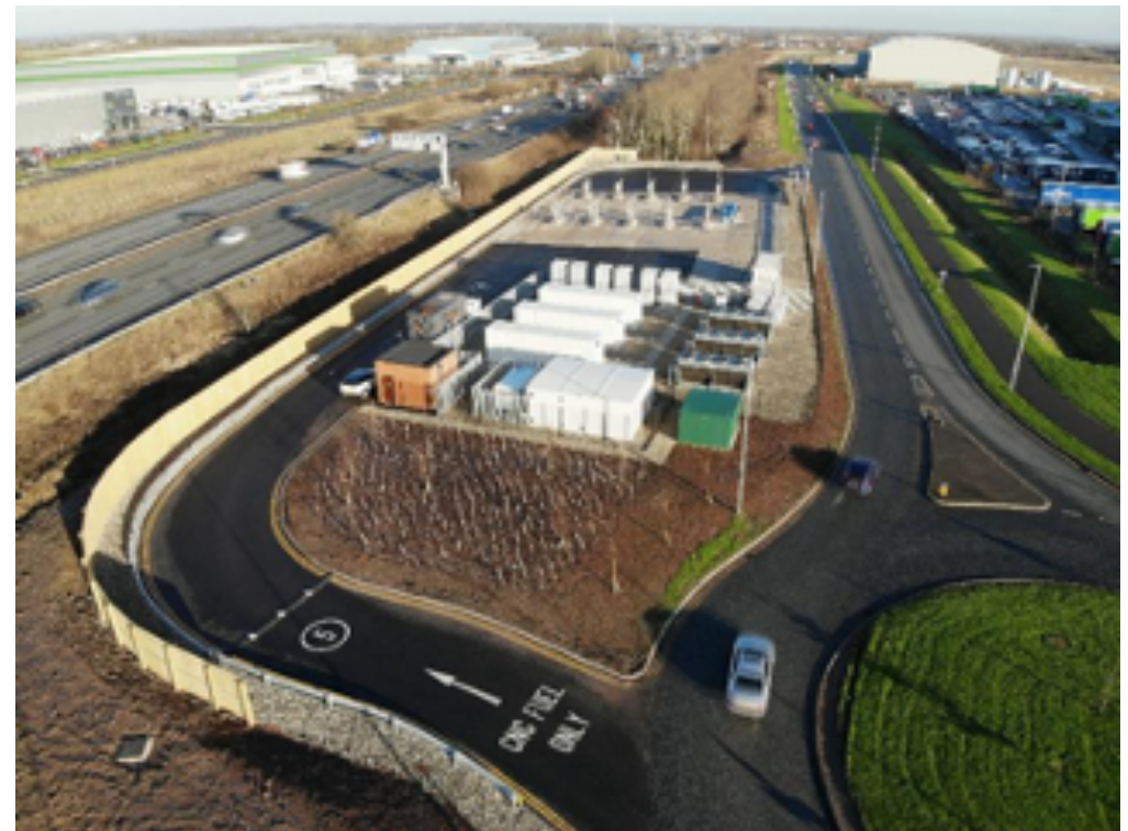
Leyland HGV NGV refuelling station. Image credit: Cadent
